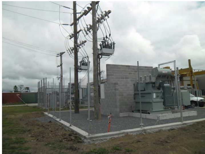
Recently Designed 33kV/11kV Private Substation for HVC
